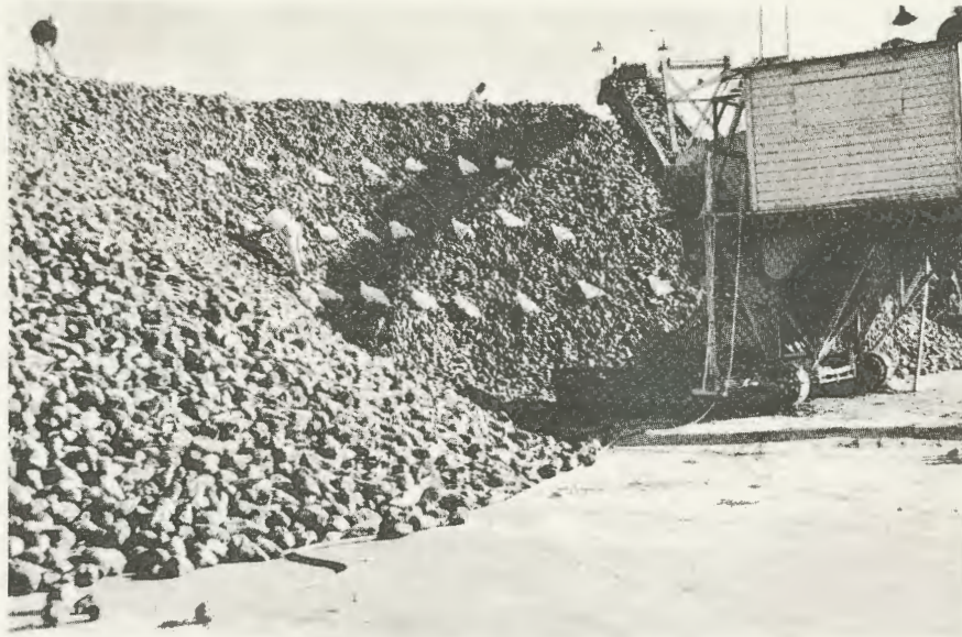
Figure 1. Captive samples in nylon mesh bags being distributed across the face of a pile to be covered by the subsequent swings of the piler boom. Nylon cords tied to the bags extend to the top of the pile where they are anchored.
